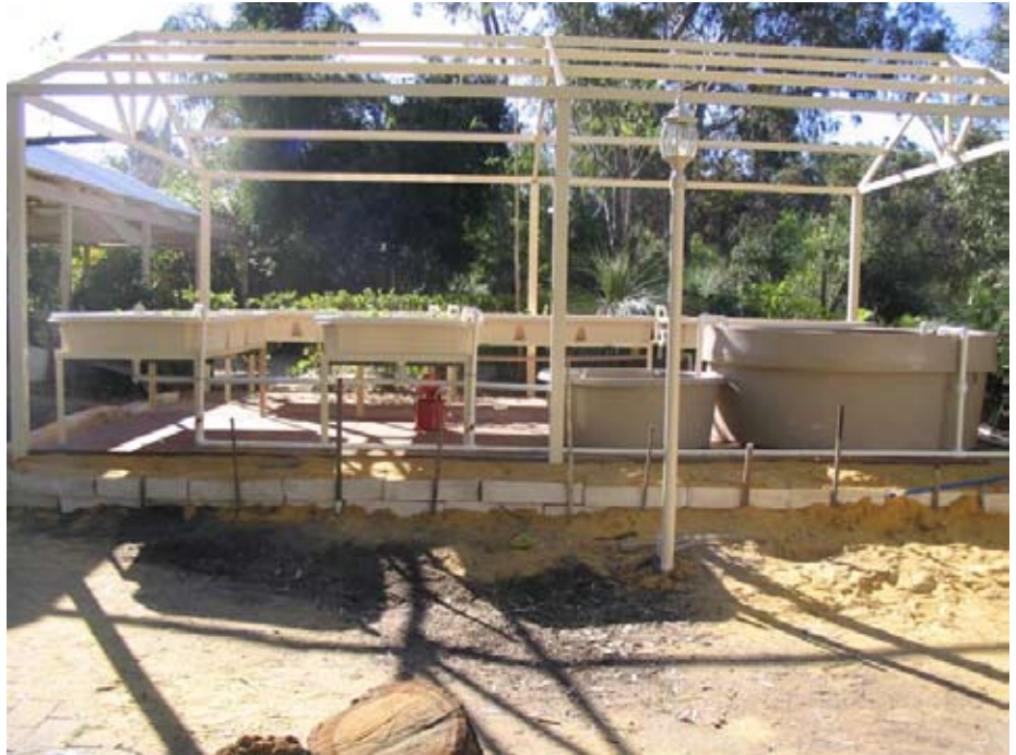
Construction work all coming together
